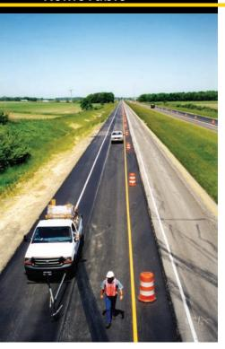
Removable pavement marking tape provides a bright, well delineated channel to guide motorists safely through construction zones and work crew areas. It is exceptionally quick and easy to install, highly durable and removes cleanly. The ideal solution to all your temporary roadway marking requirements.
